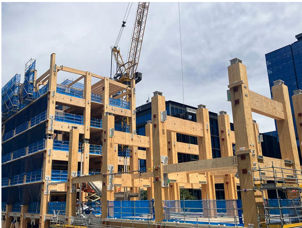
Locally manufactured CLT and LVL has replaced concrete and steel in the soon to be completed six-storey parliamentary building.
